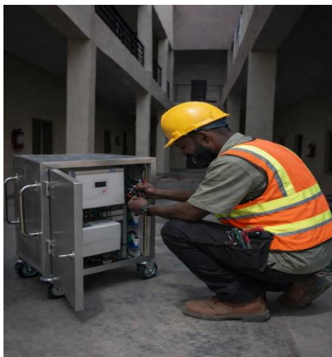
Figure 5: Battery & inverter install.
