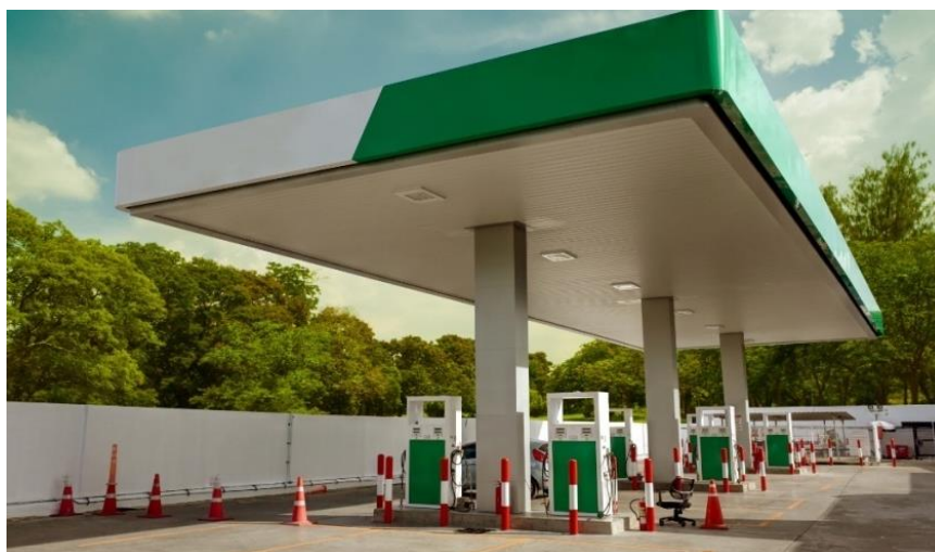
Fig. 7. - CNG Charging Station
