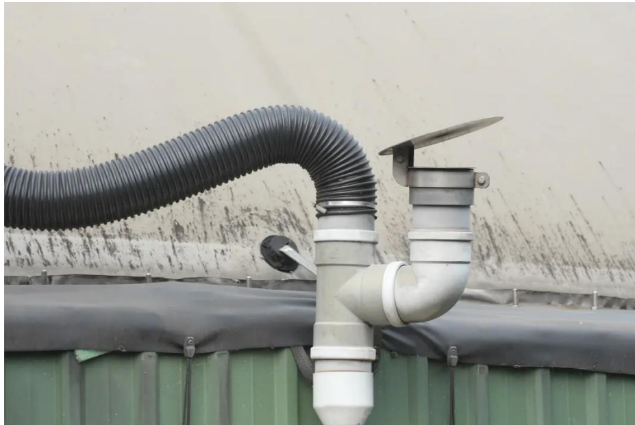
Figure 2. Biogas Leakage
