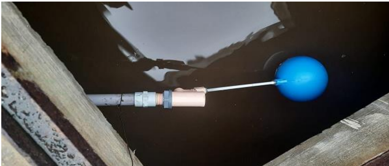
Fig 10 Float valve implementation
