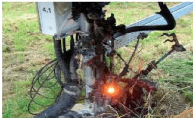
Fig. 2. Arcing persists in the DC wiring even after a fire consumes a portion of the combiner box.
