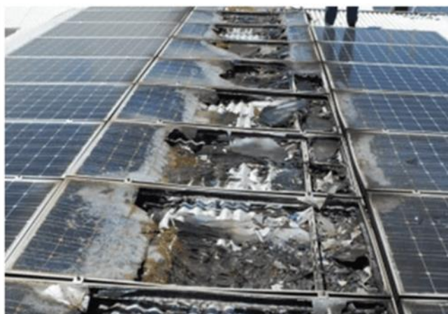
Fig. 1: Damage to a PV system attributed to an arc
