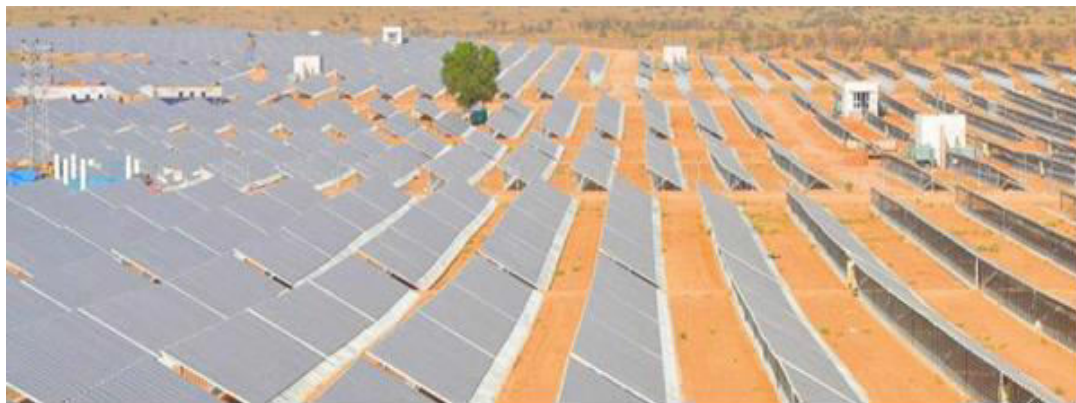
Fig 6 Shows the panels installation at Vikram Solar Limited Manchitya, Bap, Rajasthan
