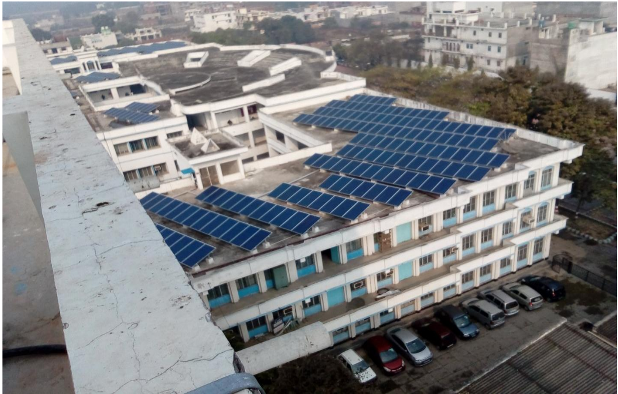
Figure : Academic Block view of Integral university Lucknow under installation process
