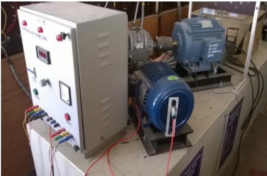
Fig. 19. Hardware setup showing the Wind turbine Emulator and PMSG.
