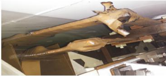
FIG 2. LV-U phase Bus bar bolted joint found affected
