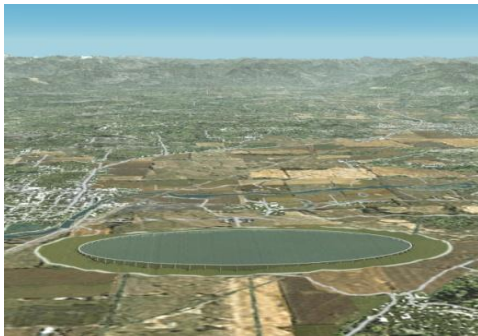
Fig.3.1 large rectenna array
