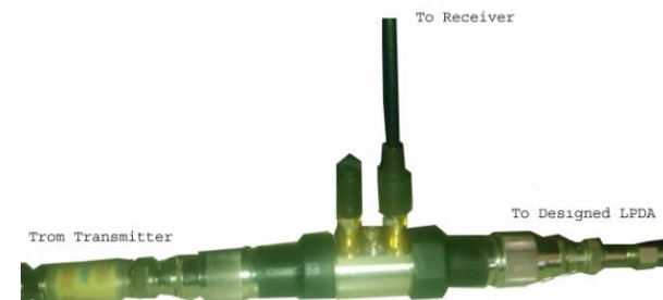
Fig.11. Connections to measure reflected power
