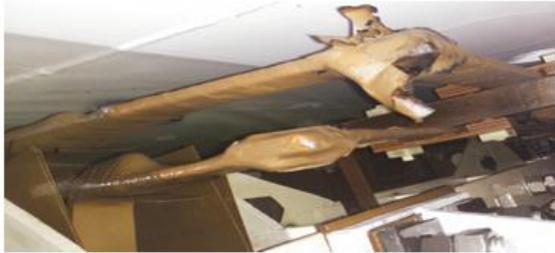
FIG 2. LV-U phase Bus bar bolted joint found affected
