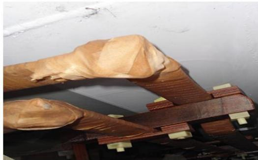
FIG 3. Paper covering and rejoining bolt
